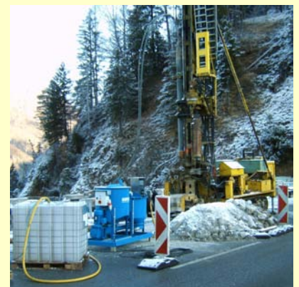
Special civil engineering Tunnel construction
